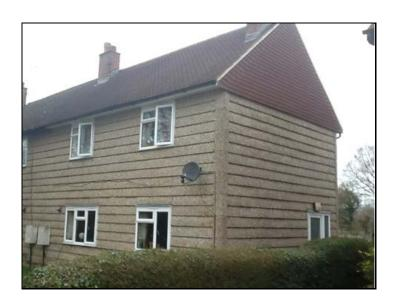
Airey's were a fast-build system to help ease the housing shortage, following WW2. Due to problems with the concrete supporting frame, they were structurally repaired, on a nation-wide scale, in the late 1980's or early 1990's. The external walls were provided with some insulation, in the form of insulated plasterboard, on the inside. Even though improved however, the thermal performance is still inferior, when compared to traditional external wall construction.
